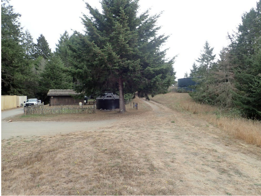
Photo 33 Water Treatment Center, view east (Marx 2020)
