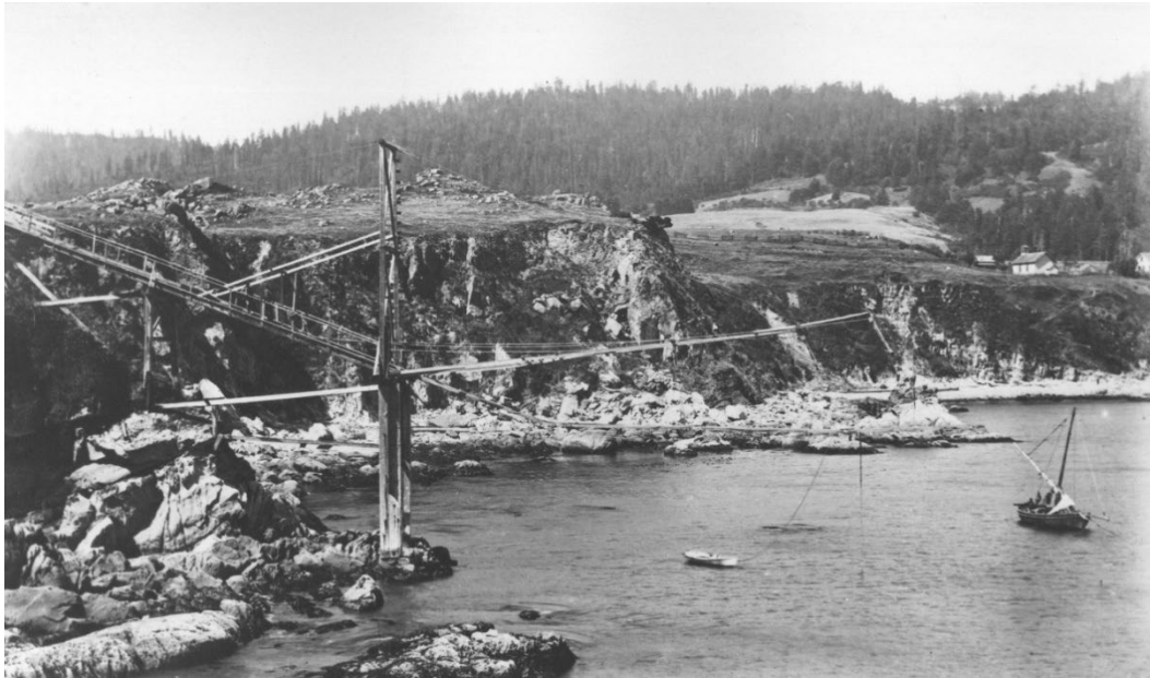
Figure 1 Trough chute at Fort Ross Landing, circa 1897 (Fort Ross Conservancy)
